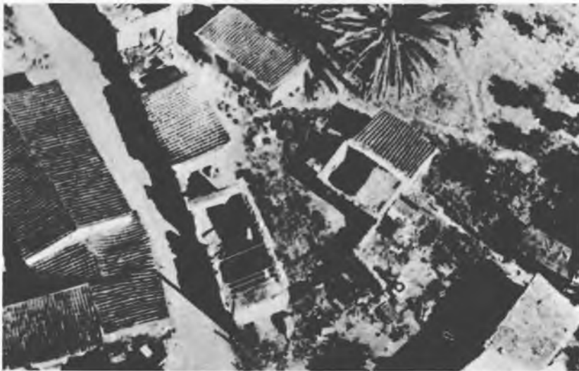
DEMOLISHED TURKISH CYPRIOT HOMES AT DHEFTERA VILLAGE
