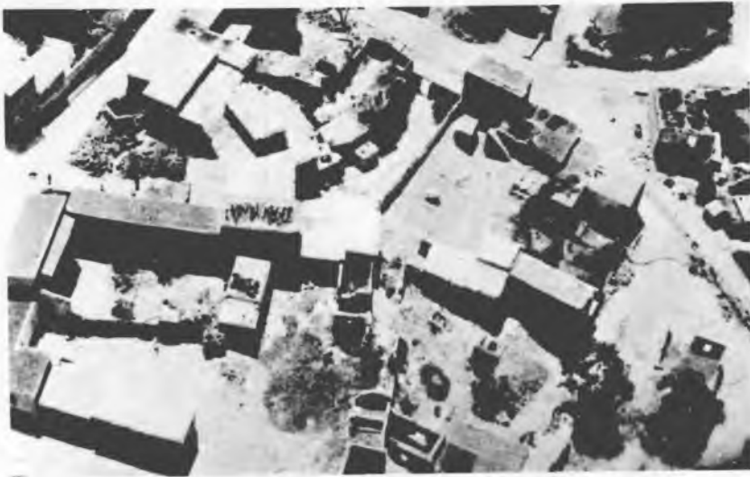
DEMOLISHED TURKISH HOUSES AT DHIORIOS VILLAGE
