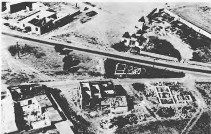
TURKISH CYPRIOT HOUSES DESTROYED AT SKYLLOURA VILLAGE
