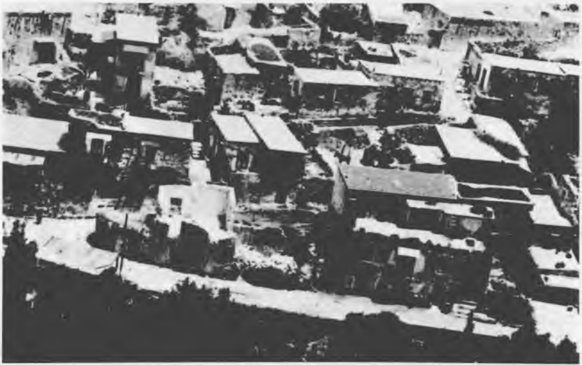
DESTROYED TURKISH CYPRIOT HOUSES AT TERRA VILLAGE
