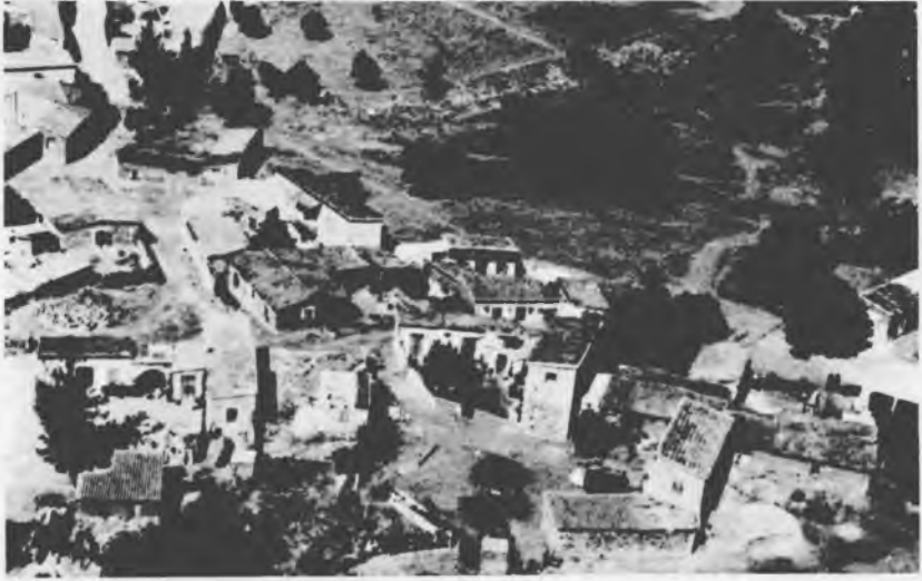
DAMAGED AND ABANDONED TURKISH CYPRIOT HOMES AT PYRGA VILLAGE
