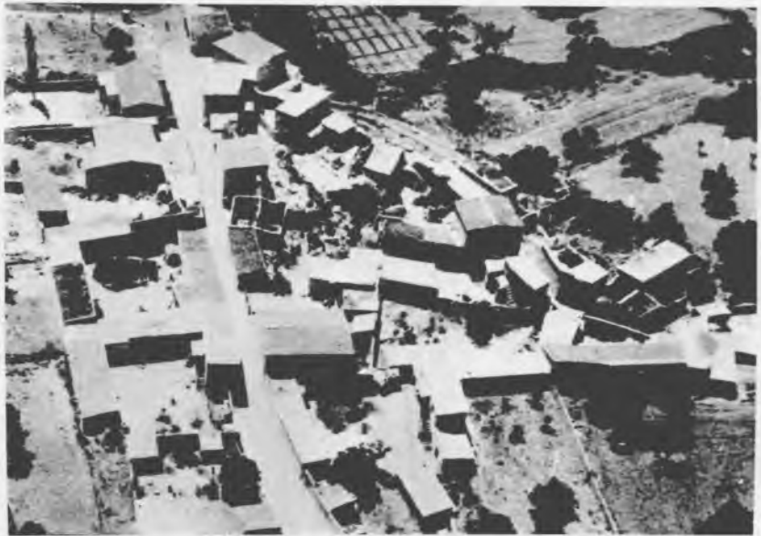
DEMOLISHED TURKISH CYPRIOT HOUSES AT ALETHRIKO VILLAGE
